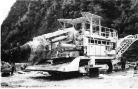
Fig. 2: Road Header PAURAT-242 after commissioning
